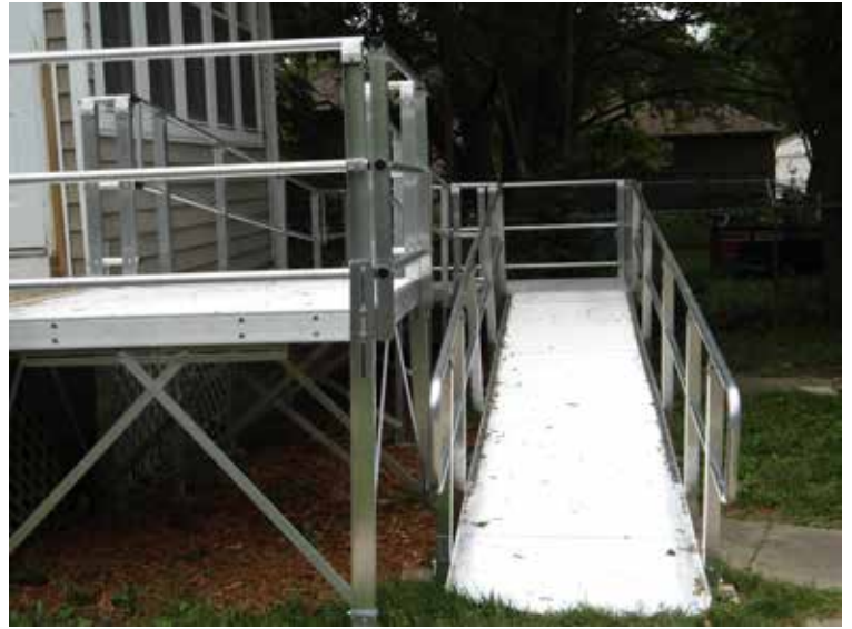
A finished ramp.
